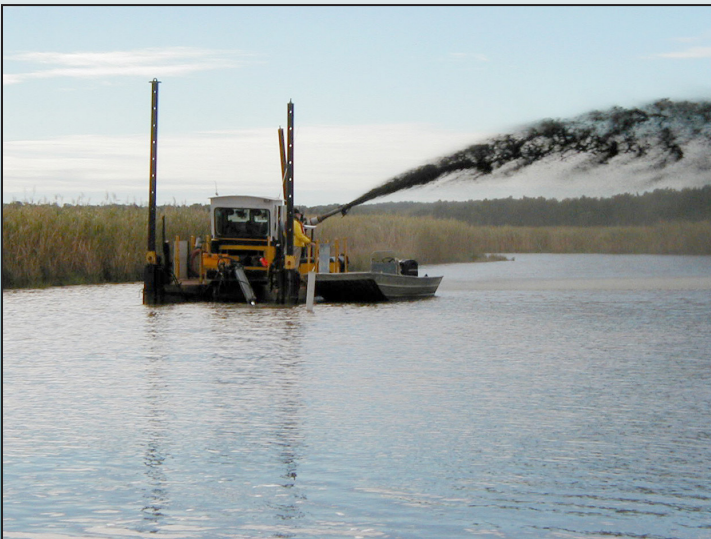
Thin-layer application of dredge material on a salt marsh in the Pamunkey River, Virginia. Photo credit: Carlton Hershner, VIMS.
