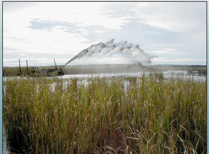
Thin-layer application of dredge material on a salt marsh in the Pamunkey River, Virginia. Photo credit: Carlton Hershner, VIMS.
